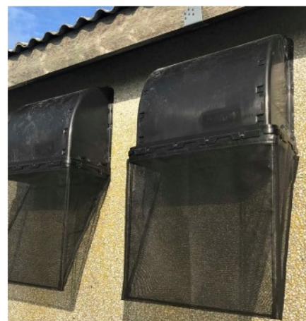
DA 1200 inlets with inlet cover and fly screen
