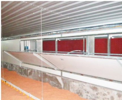
Rack & Pinion as the tunnel door solution in a tunnel ventilated house
