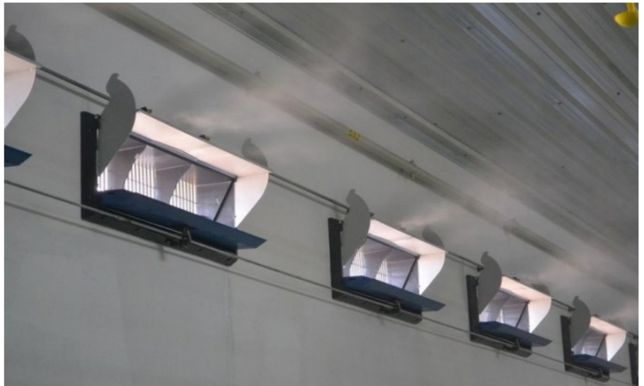
DA 1911 inlet with long air direction baffle
