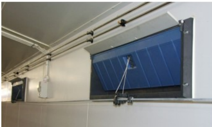
DA 1911 inlet with short air direction baffle
