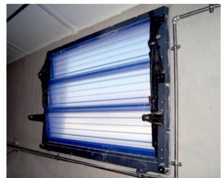
The DA 10K with transparent flaps when outdoor light is required
