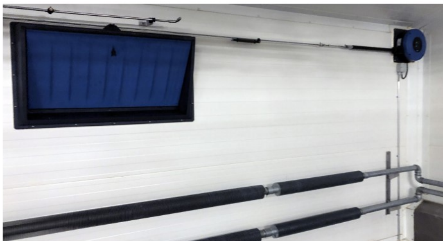
The DA 175 with the DA 3800 wall inlet in a simple setup
