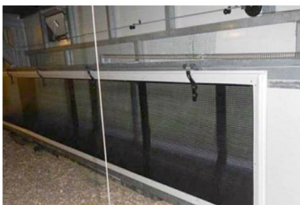
Tunnel Door Light closing system for houses with Tunnel or Combi-Tunnel.
