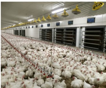
DA 17K as tunnel doors in a Combi-Tunnel broiler house
