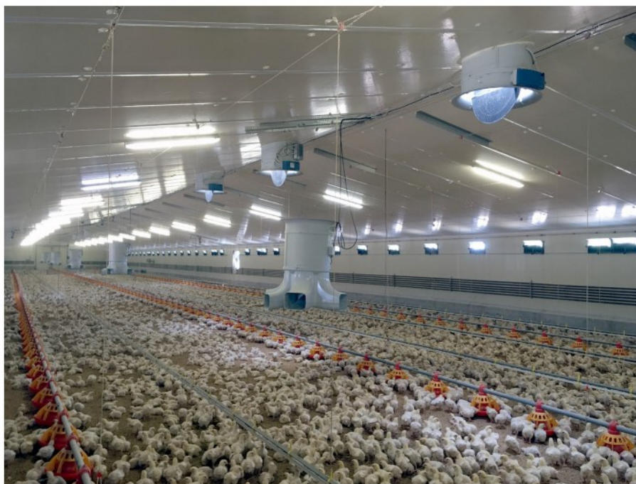
DA 65-600 chill units working together with DA 1911 inlets to ensure a pleasant floor level climate.
