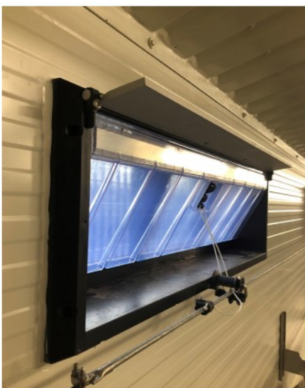
DA 1911 inlet with transparent flap for light access
